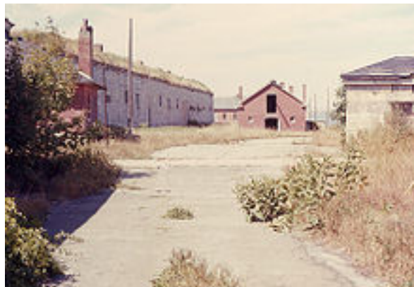
A section of historic Fort Adams in a neglected state (1968)
